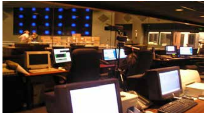
Command and Control Facilities
