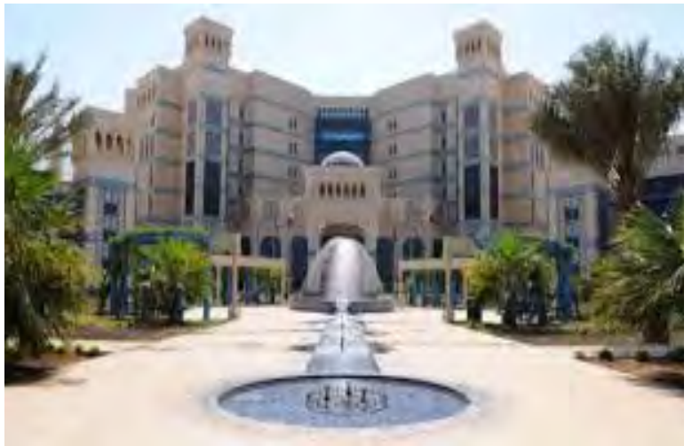
Al Wakra Hospital - Qatar
