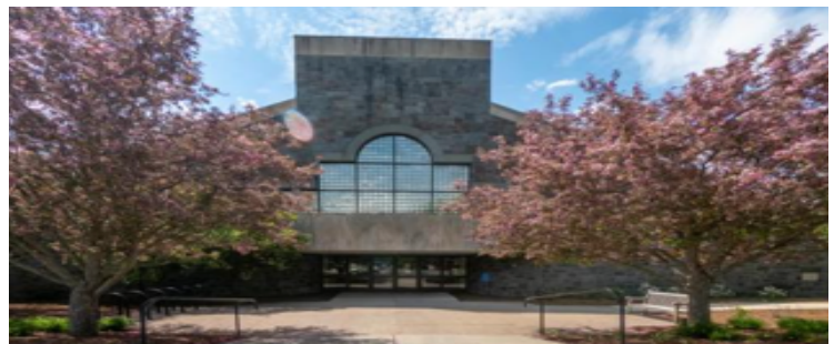
Sanford Fieldhouse - Security Alterations
